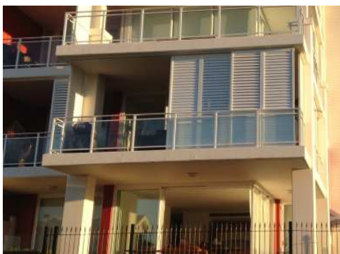
Image 2. Adjustable louvre screen on balcony.
