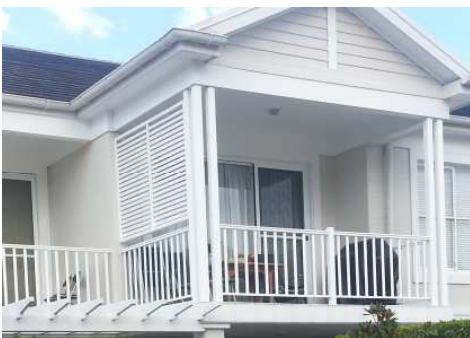
Image 1. Slatted timber screen on the side of balcony.
